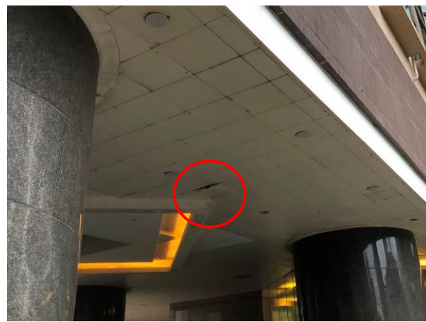
Photo No. C68 Damaged ceiling panel forming gap.
