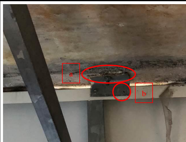
Photo No. C26 a) GMS plate was rusty. b) Screws were missed.
