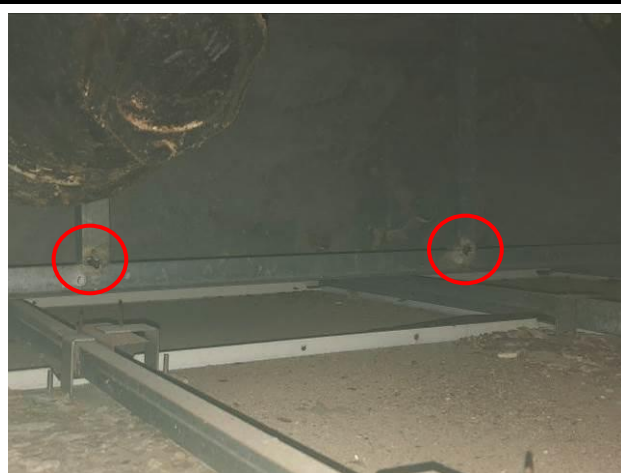
Photo No. C53 | Welded joints were rusty.
