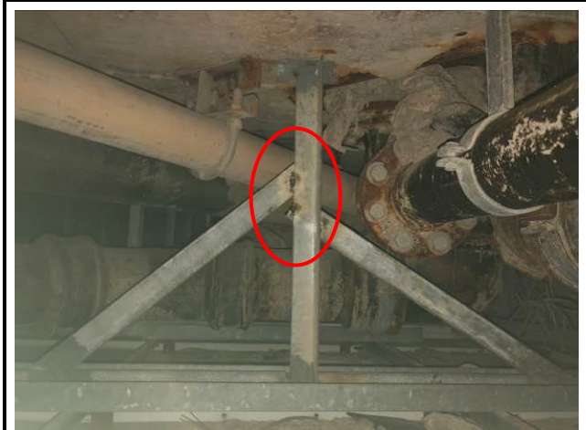
Photo No. C12 | Welded joints were rusty.
