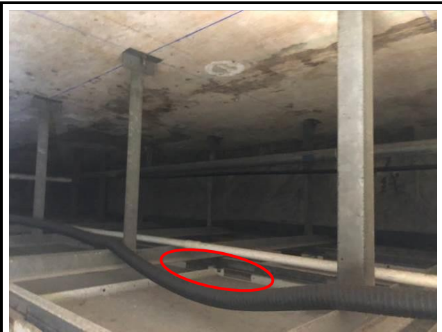
Photo No. B44 Brackets connecting grid and ceiling panel were rusty.
