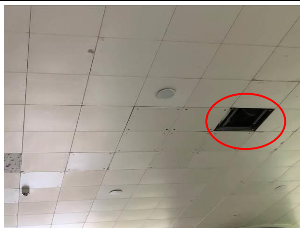
Photo No. A41 | 1 piece of ceiling panel was missing.
