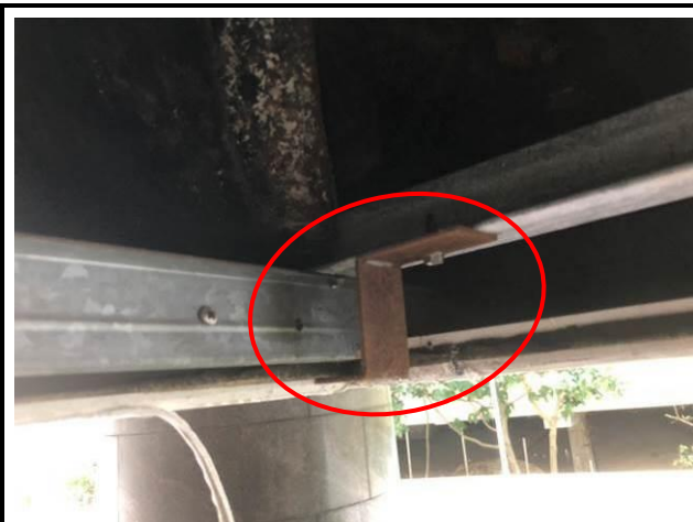
Photo No. A45 | Bracket connecting grid and access panel was rusty.
