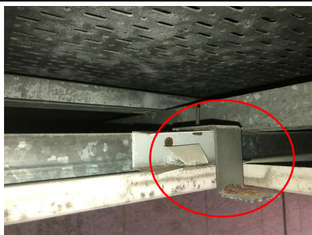
Photo No. C58 Bracket connecting grid and access panel and screws were rusty.
