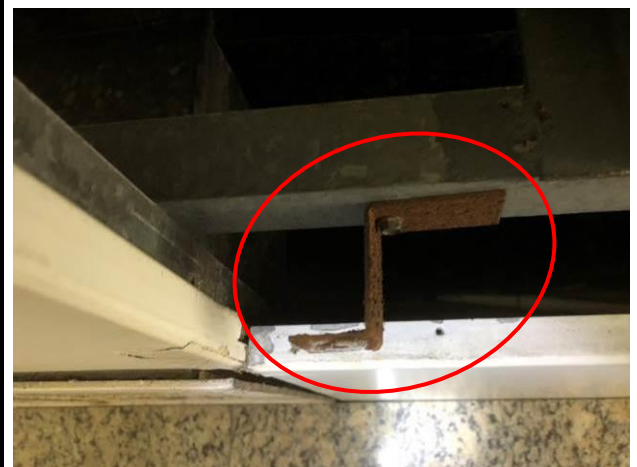
Photo No. A40 | Bracket connecting grid and access panel was rusty.
