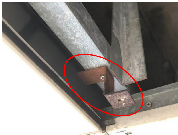
Photo No. C13 Bracket connecting grid and access panel was rusty.
