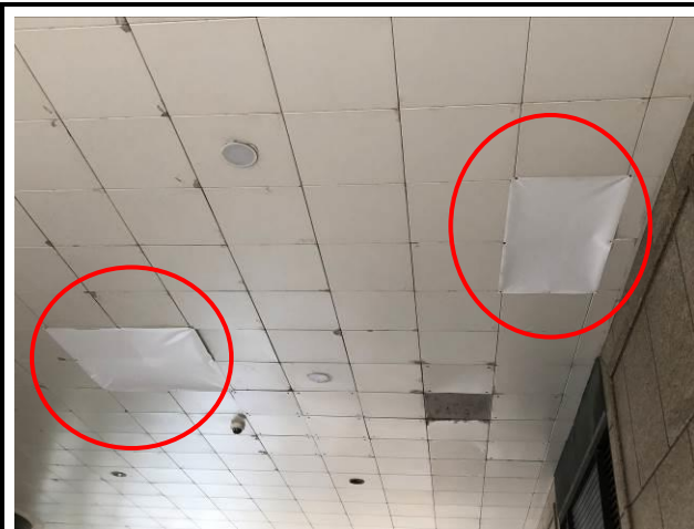
Photo No. C43 | 6 pieces of ceiling panels were missing.
