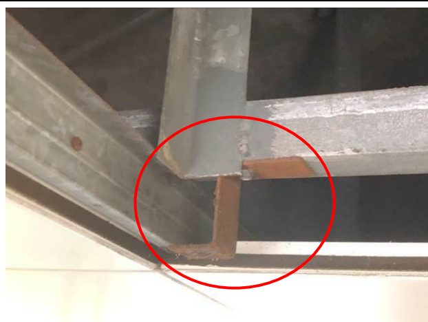
Photo No. A15 | Bracket connecting grid and access panel was rusty.
