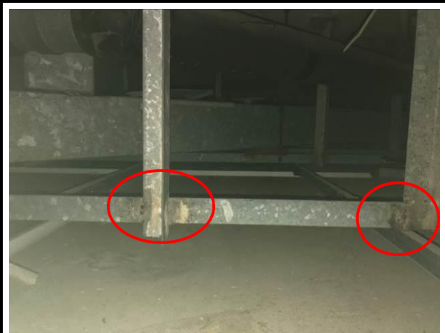
Photo No. B26 | Welded joints were rusty.
