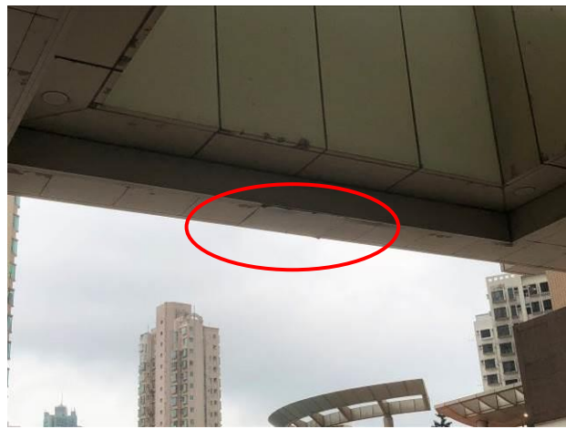
Photo No. B55 | 2 pieces of ceiling panel were missing.
