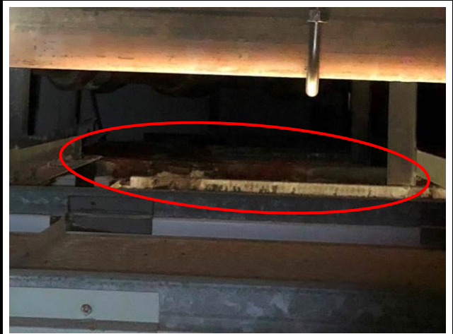
Photo No. A34 | Ceiling grid was rusty.
