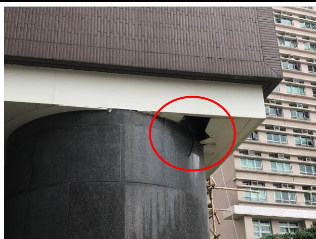
Photo No. A27 1 piece of ceiling panel was missing
