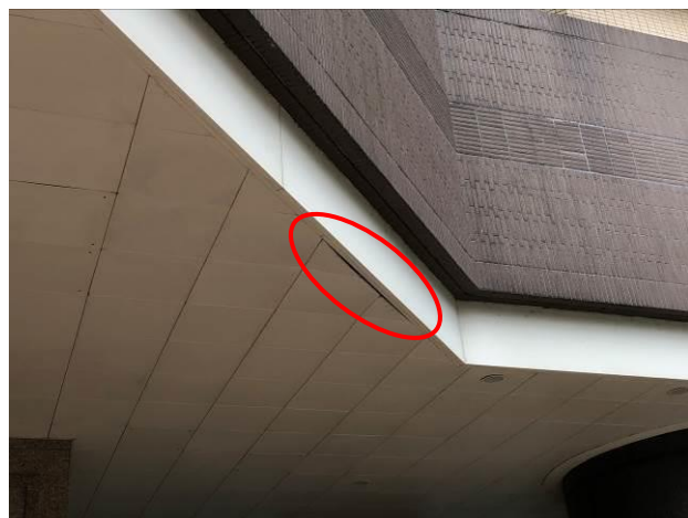
Photo No. A13 | Damaged ceiling panels forming gap.
