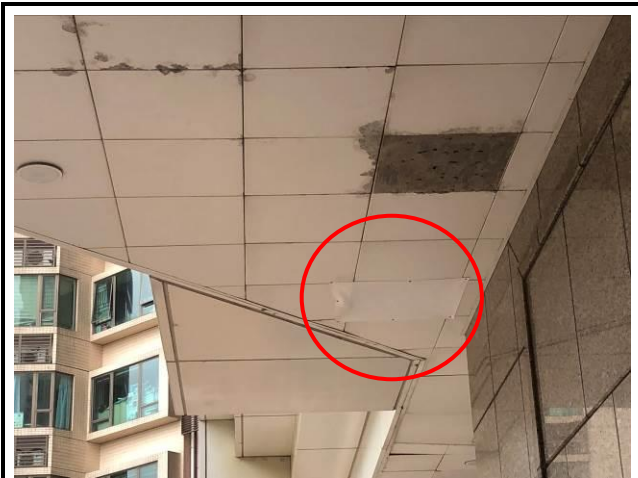
Photo No. C44 | 1 piece of ceiling panel was missing.
