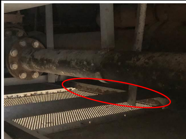
Photo No. B36 | Ceiling grid was rusty.
