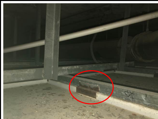
Photo No. C47 | Bracket connecting grid and ceiling panel was rusty.
