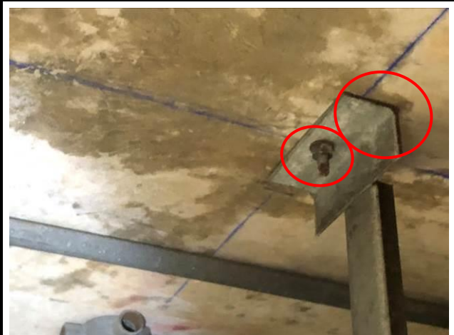
Photo No. B46 a) Bolt was rusty. b) Edge of GMS plate was rusty.
