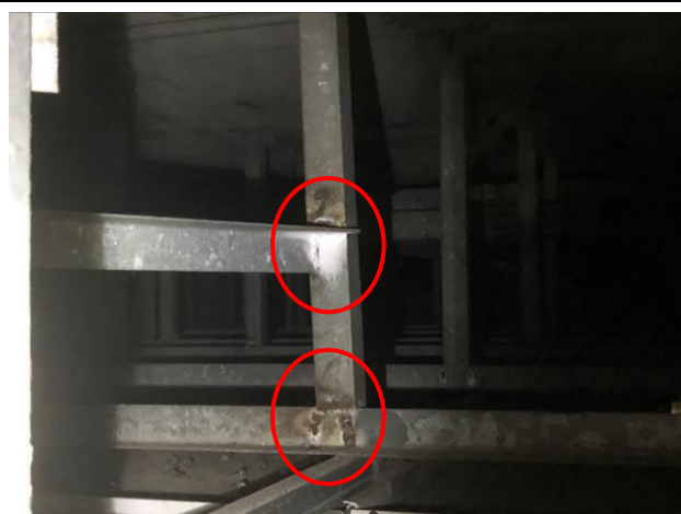
Photo No. A17 | Welded joints were rusty.
