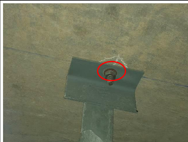
Photo No. B22 Washer plate was rusty.
