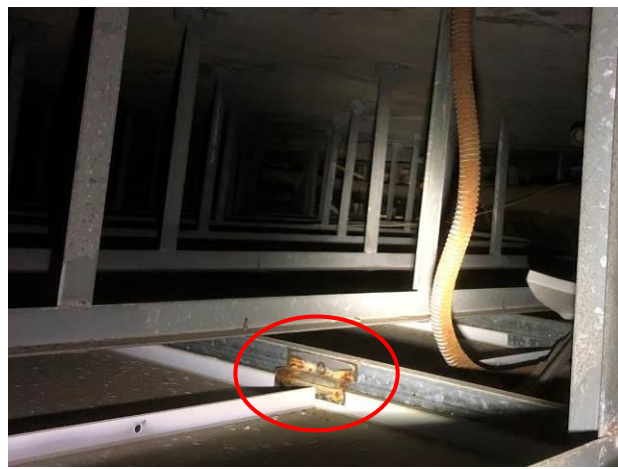
Photo No. A37 | Bracket connecting grid and ceiling panel was rusty.
