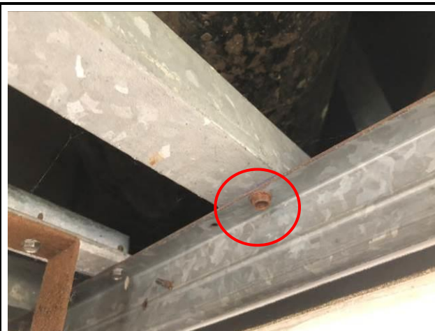
Photo No. A46 | Screw was rusty.
