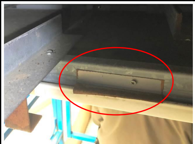
Photo No. B6 | Bracket connecting grid and ceiling panel was rusty.
