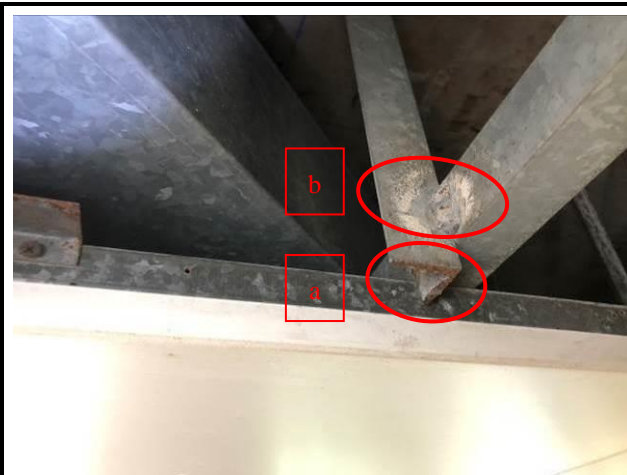
Photo No. B29 | a) Edge of GMS post was rusty. b) Welded joints were rusty.
