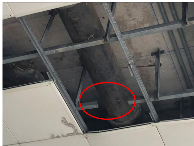
Photo No. C31 | Ceiling grid was discrete.
