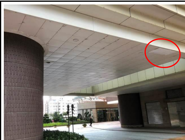
Photo No. B49 | 2 pieces of ceiling panel were missing.
