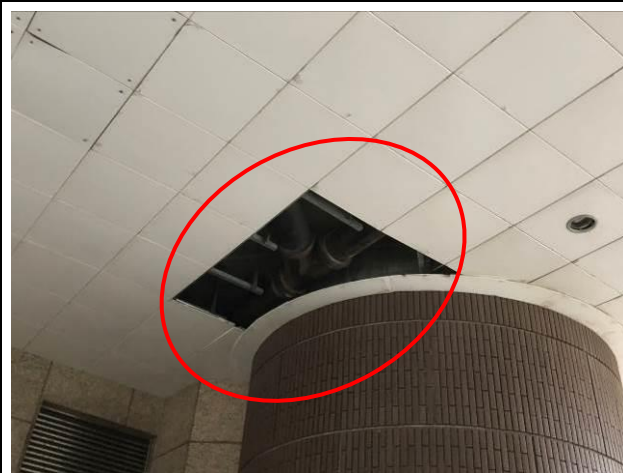
Photo No. B54 | 5 pieces of ceiling panel were missing.
