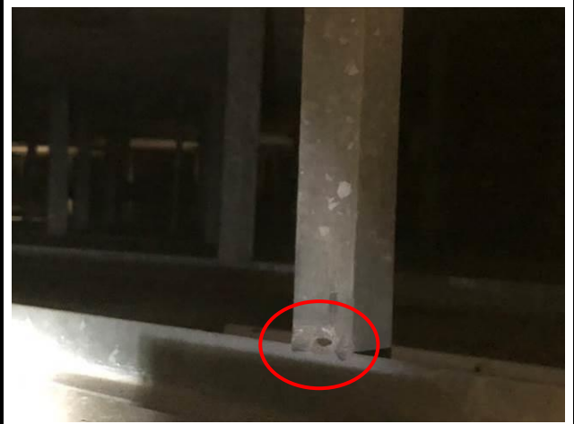
Photo No. A32 | Hole was found on weld joint.
