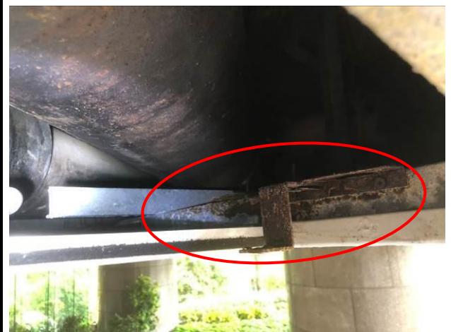
Photo No. B58 | Ceiling grid and bracket were rusty.
