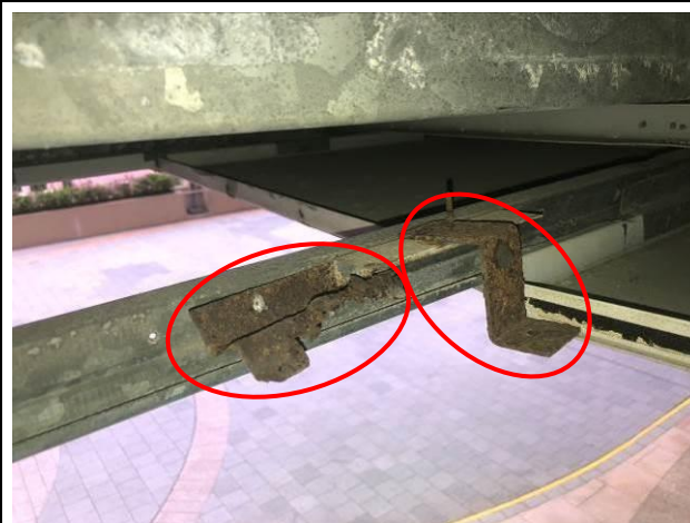
Photo No. C34 | Brackets connecting grid and access panel/ panels were rusty and corroded.
