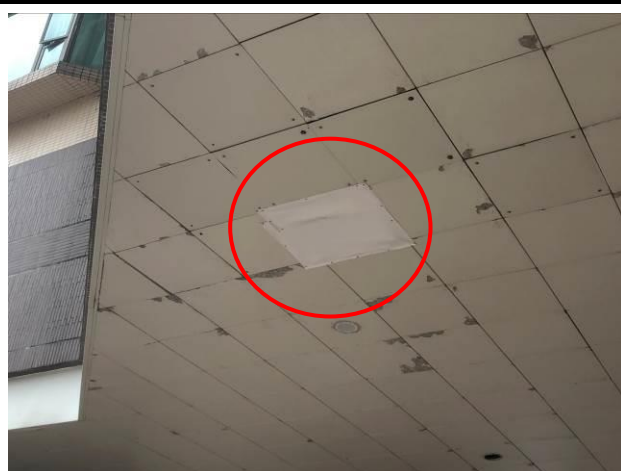
Photo No. C41 | 1 piece of ceiling panel was missing.
