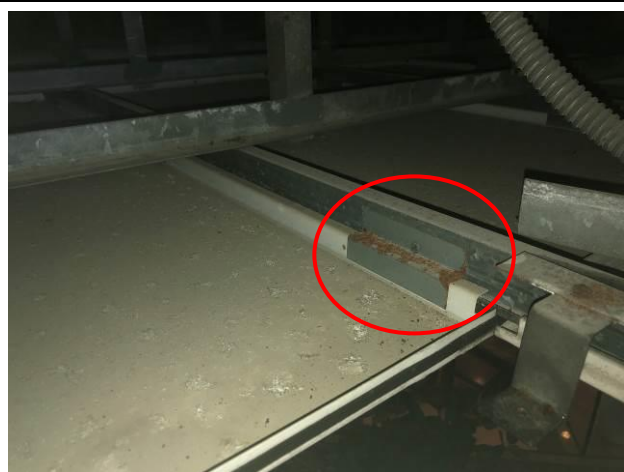
Photo No. C63 | Bracket connecting grid and access panel was rusty.
