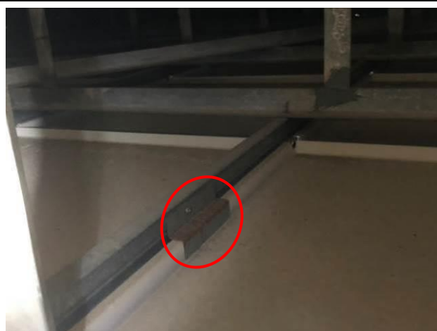
Photo No. C5 | Bracket connecting grid and ceiling panel was rusty.
