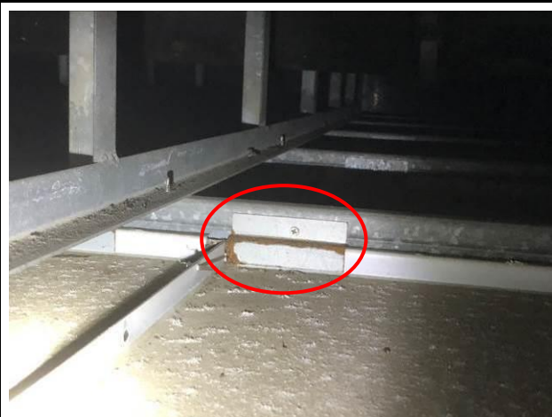
Photo No. A22 | Bracket connecting grid and ceiling panel was rusty.
