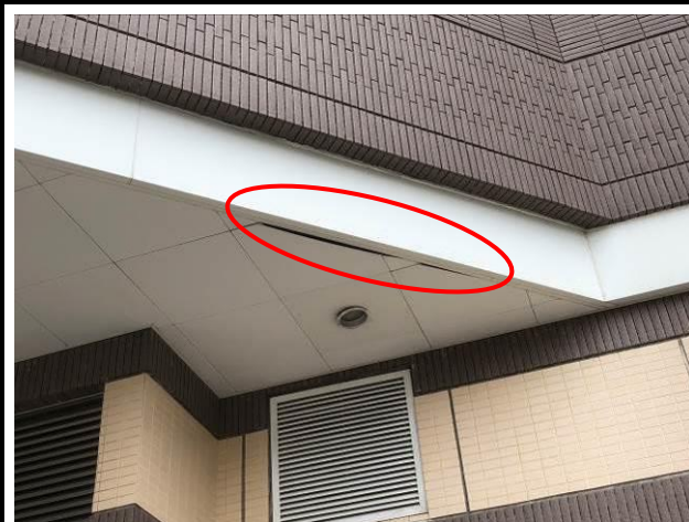
Photo No. A6 | Damaged ceiling panels forming gap.
