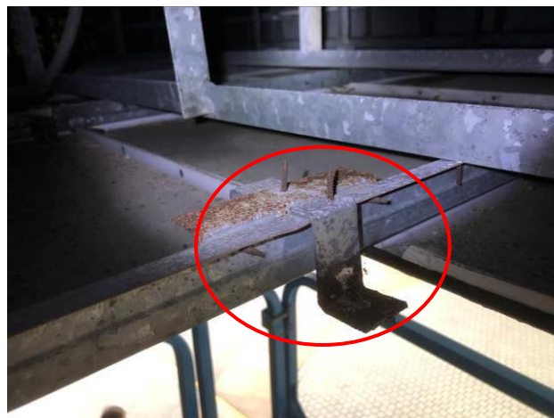
Photo No. C55 Bracket connecting grid and access panel was rusty.
