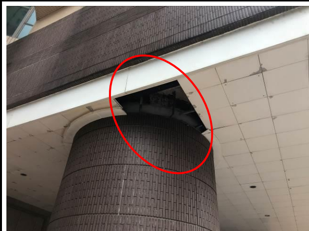
Photo No. C27 4 pieces of ceiling panels were missing.
