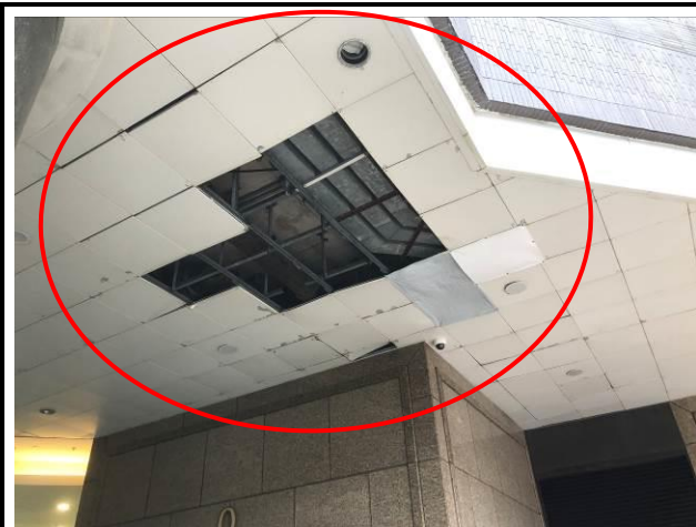
Photo No. C29 13 pieces of ceiling panel were missing and the surrounding panels were loosening.
