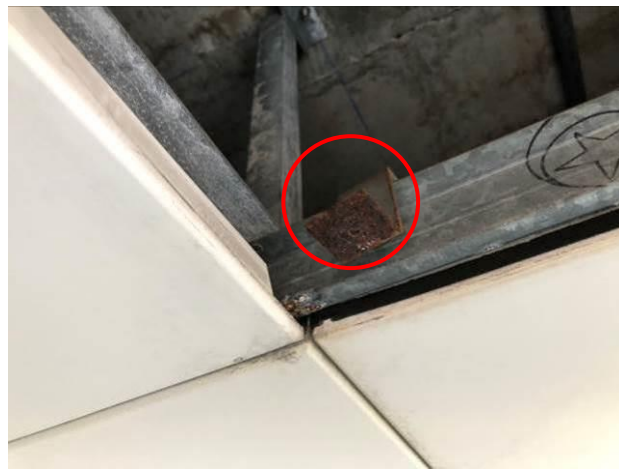
Photo No. C7 | Bracket connecting grid and access panel was rusty.
