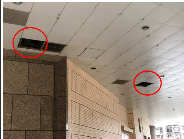
Photo No. C14 2 pieces of ceiling panels were missing.
