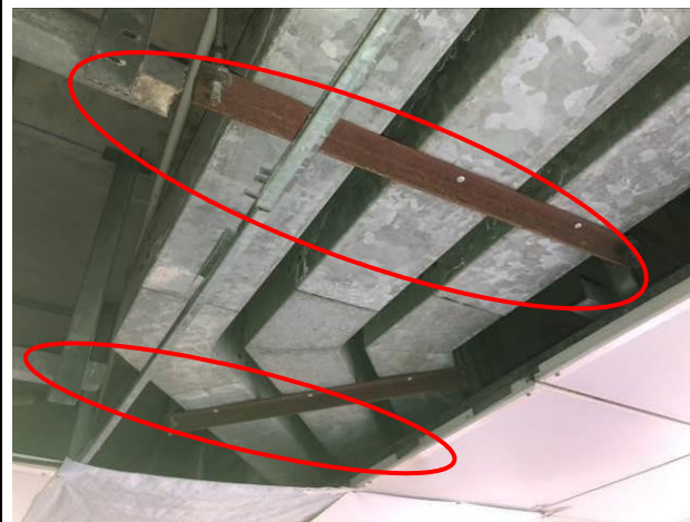
Photo No. C32 | Ceiling grids were discrete.
