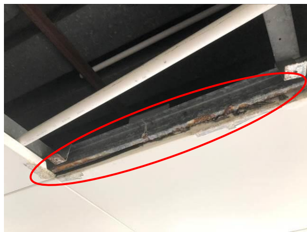
Photo No. B37 | Ceiling grid was rusty.
