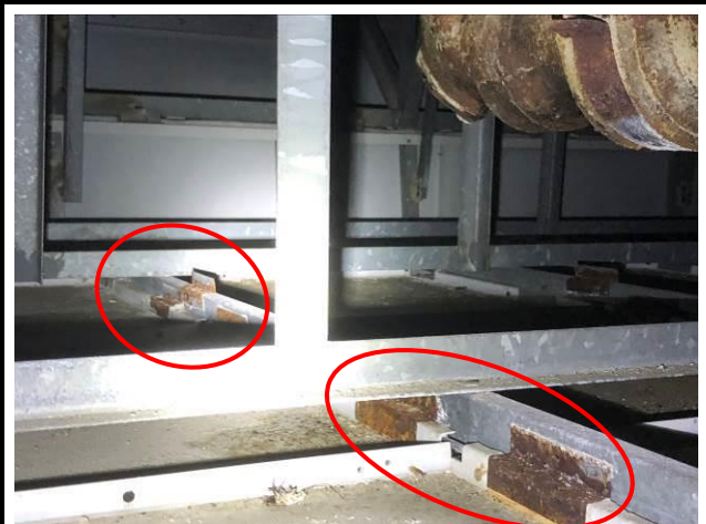
Photo No. C54 | Brackets connecting grid and ceiling panel were rusty.
