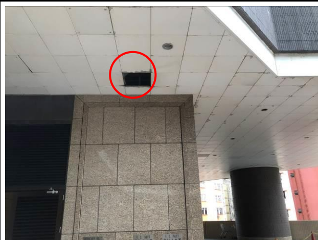
Photo No. C28 1 piece of ceiling panel was missing.
