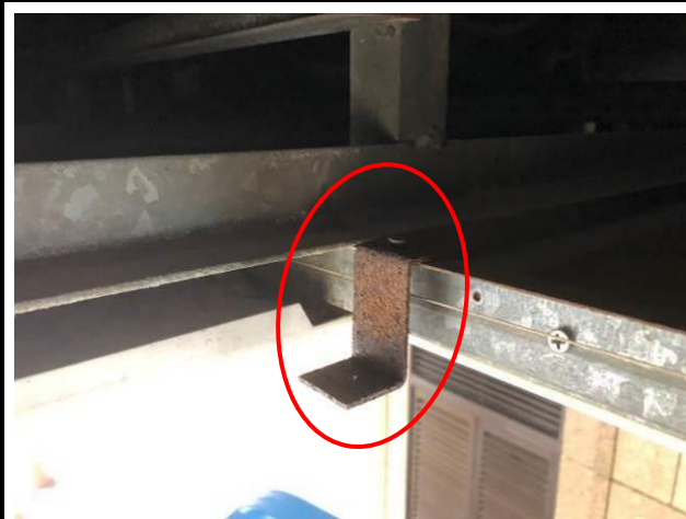
Photo No. C19 Bracket connecting grid and access panel was rusty.
