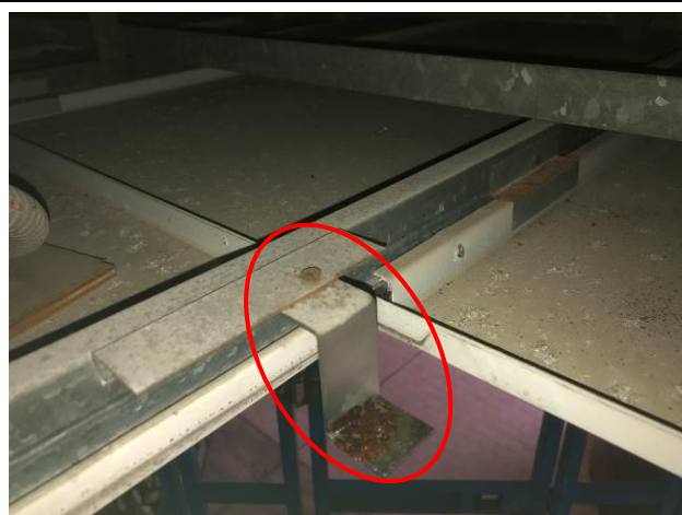
Photo No. C65 | Bracket connecting grid and access panel and screw were rusty.
