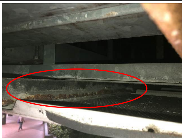
Photo No. C59 Ceiling grid was rusty.
