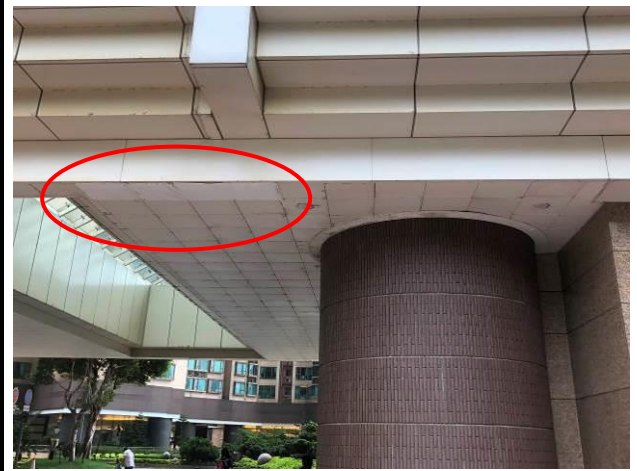
Photo No. C50 | 4 pieces of ceiling panels were missing.
