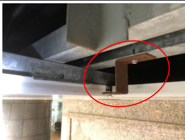
Photo No. A29 Bracket connecting grid and access panel was rusty.
