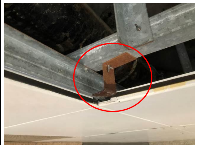
Photo No. A12 | Bracket connecting grid and access panel was rusty.
