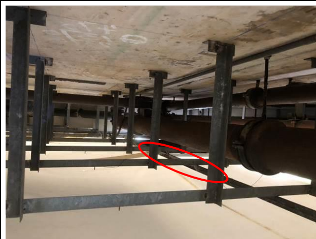
Photo No. B42 | Ceiling grid was rusty.
