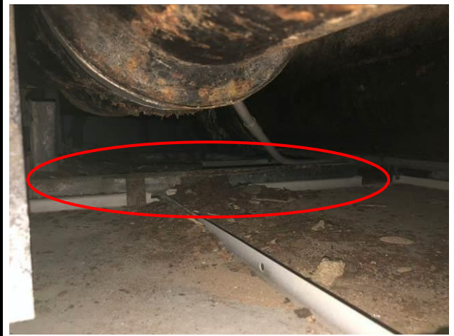
Photo No. C38 | Ceiling grid was rusty.
