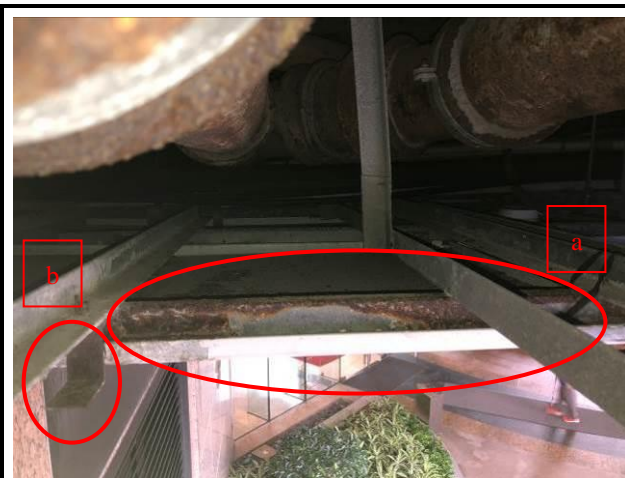
Photo No. B14 a) Ceiling grid was rusty. b) Bracket connecting grid and access panel was rusty.
