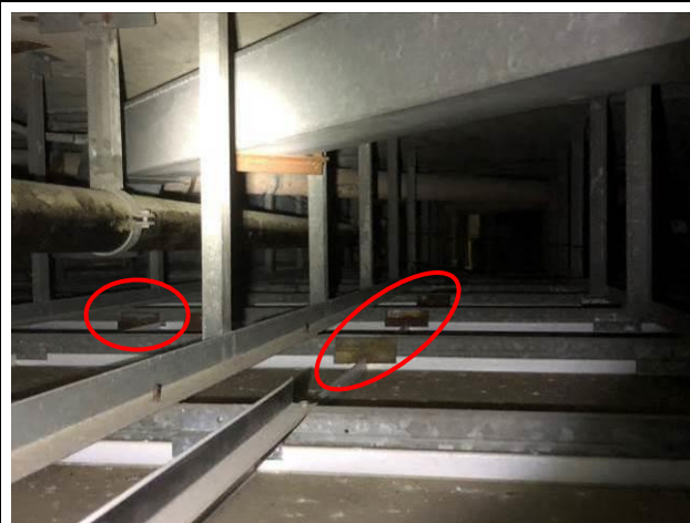
Photo No. B20 Brackets connecting grid and ceiling panel were rusty.
