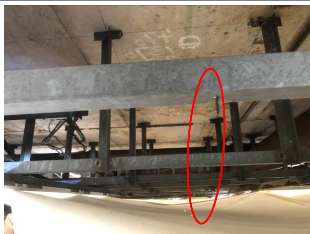
Photo No. B39 | Ceiling grids were damaged with screws remaining.
