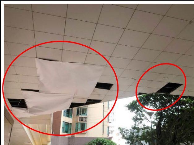
Photo No. B47 45 pieces of ceiling panel were missing.
