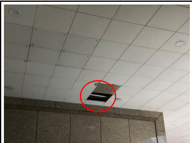
Photo No. B30 | 1 piece of ceiling panel was missing
