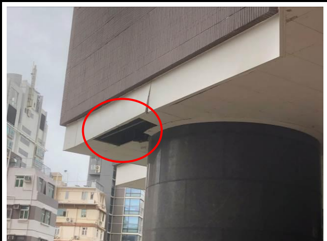
Photo No. C42 | 3 pieces of ceiling panels were missing.
