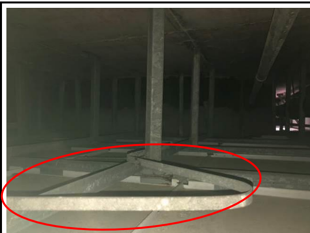
Photo No. C22 Debris/ unused materials were found on panels.
