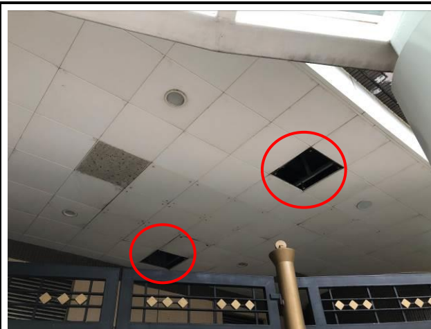
Photo No. A48 | 2 pieces of ceiling panels were missing.
