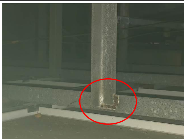
Photo No. B19 Welded joints were rusty.
