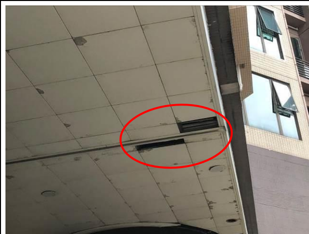
Photo No. B68 | 2 pieces of ceiling panel were missing.
