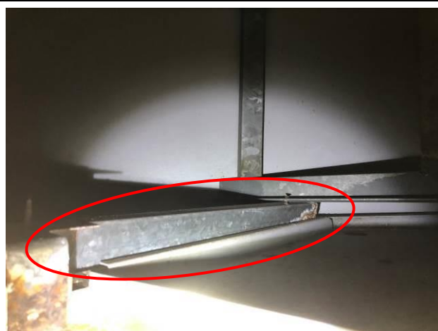
Photo No. B59 | Ceiling grid was inclined and rusty.
