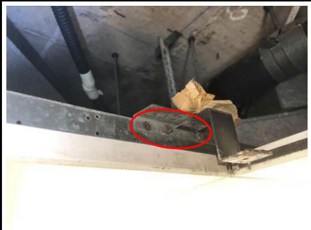
Photo No. B28 | Screws were rusty
