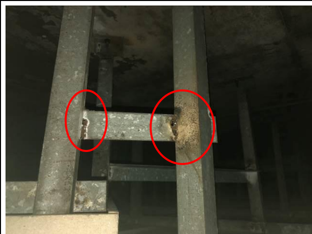
Photo No. A16 | Welded joints were rusty.
