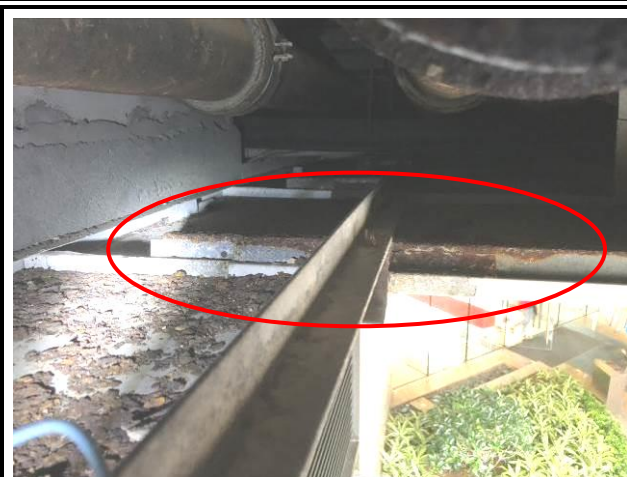
Photo No. B15 Ceiling grid was rusty.
