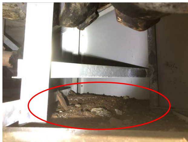
Photo No. B57 | Debris was found on ceiling panels.
