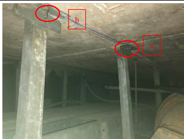
Photo No. C33 | a) GMS plate was rusty. b) Bolt was rusty.
