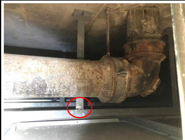
Photo No. B53 | Welded joints were rusty.
