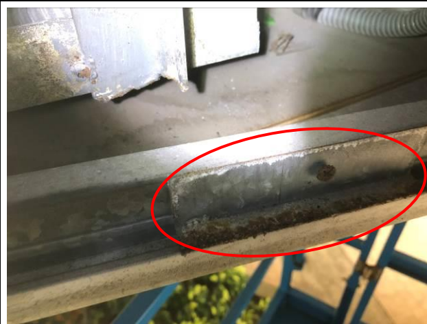
Photo No. C64 | Bracket connecting grid and access panel and screw were rusty.
