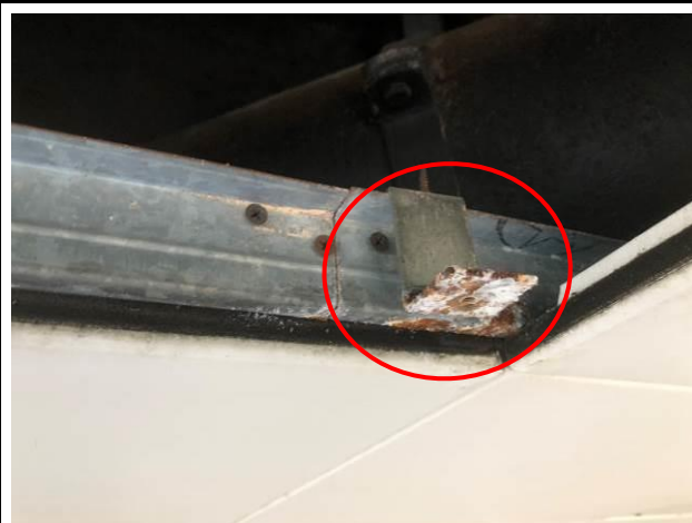
Photo No. B64 | Bracket connecting grid and access panel was rusty.
