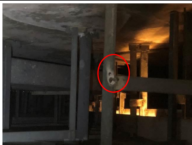
Photo No. A19 | Welded joints were rusty.
