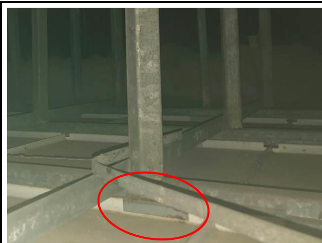
Photo No. C23 Bracket connecting grid and ceiling panel was rusty.
