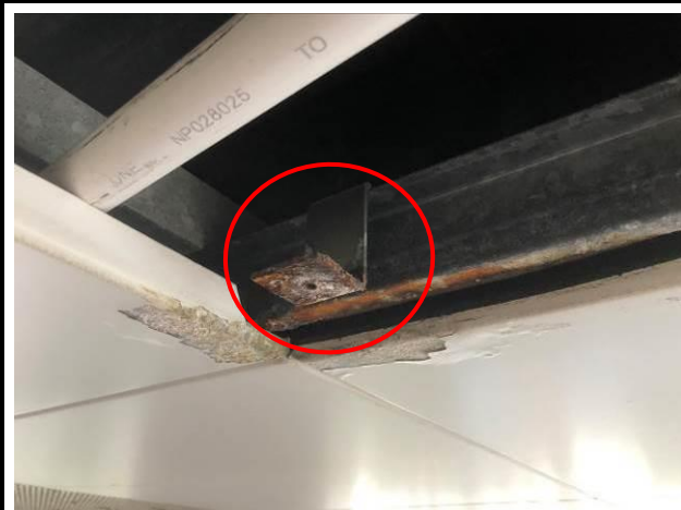
Photo No. B34 | Bracket connecting grid and access panel was rusty.
