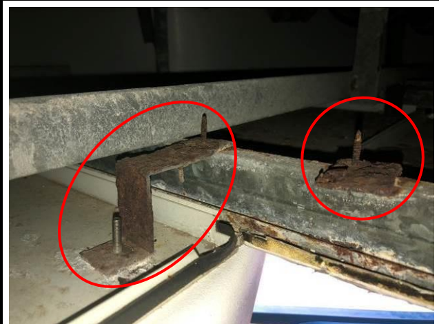
Photo No. C40 | Brackets connecting grid and access panel were rusty.
