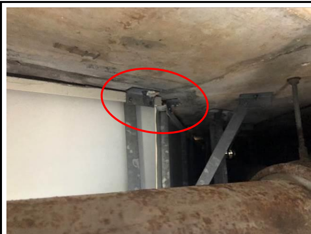
Photo No. C24 GMS plates were rusty.
