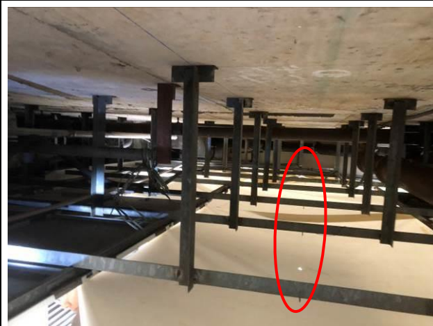
Photo No. B40 | Ceiling grids were damaged with screws remaining.
