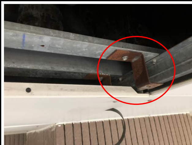
Photo No. B5 | Bracket connecting grid and access panel was rusty.
