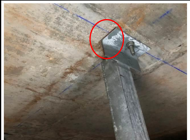
Photo No. C6 | Edge of GMS plate was rusty
