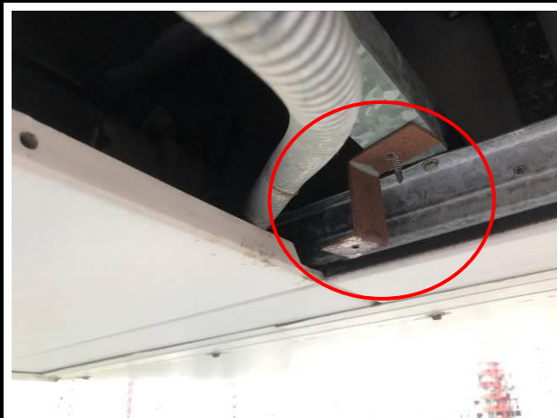
Photo No. A4 | Bracket connecting grid and access panel was rusty.
