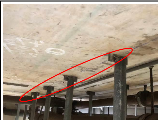
Photo No. B43 Welded joints were rusty.
