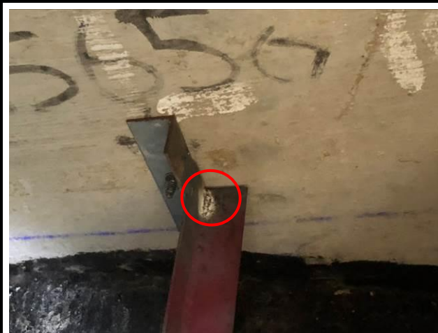
Photo No. B25 | Welded joints were rusty.
