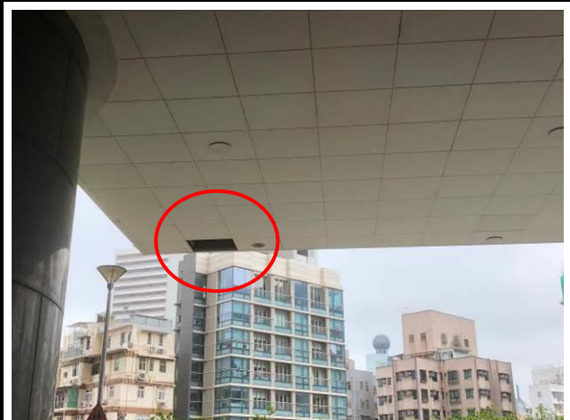
Photo No. B48 1 piece of ceiling panel was missing.
