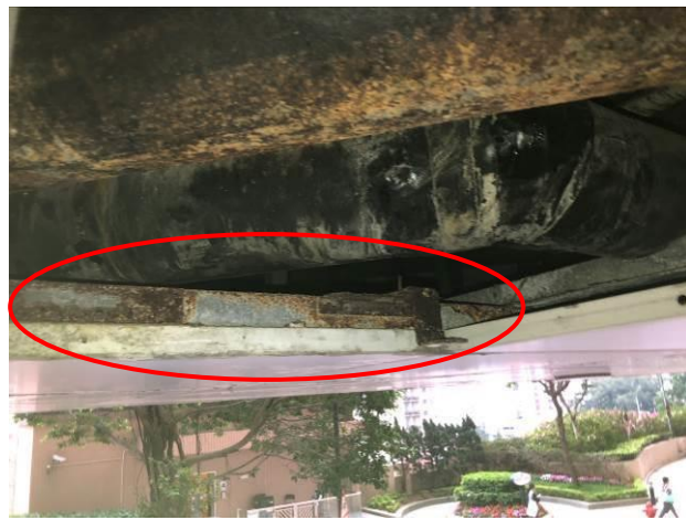
Photo No. C49 | Ceiling grid was rusty.
