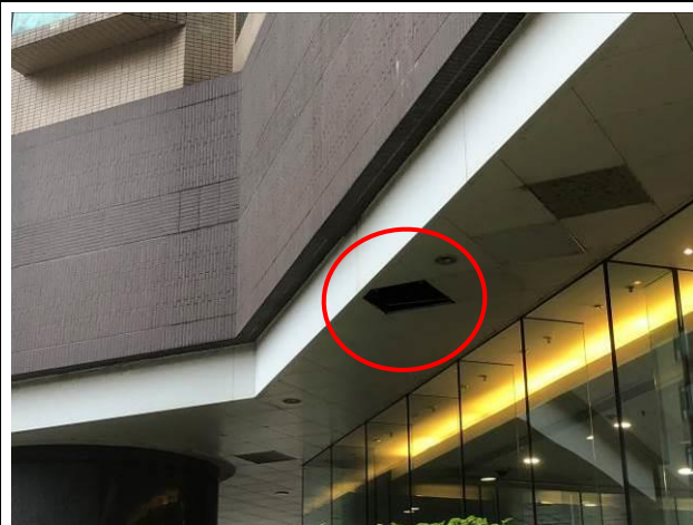
Photo No. B66 | 1 piece of ceiling panel was missing.
