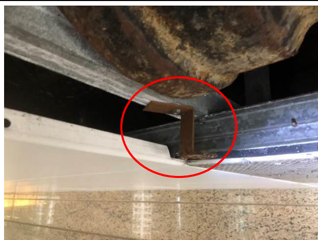
Photo No. A25 Bracket connecting grid and access panel was rusty.
