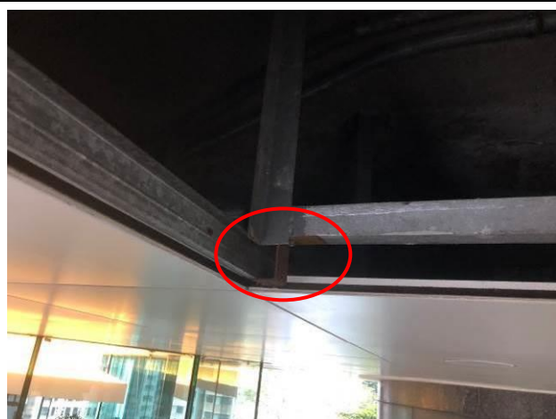
Photo No. B23 Bracket connecting grid and access panel was rusty.
