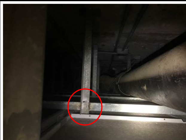
Photo No. A24 | Welded joints were rusty.
