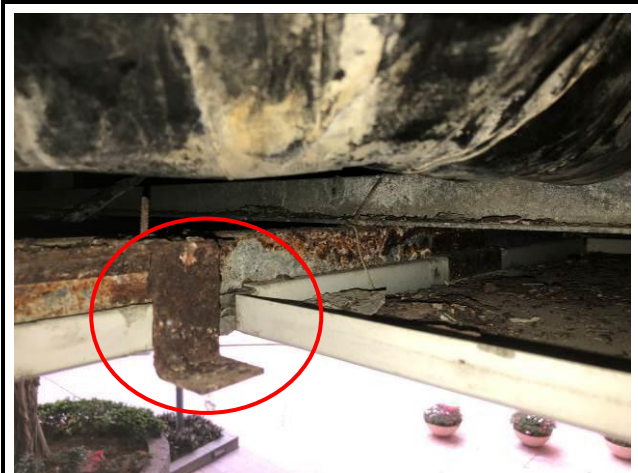
Photo No. C48 | Bracket connecting grid and access panel was rusty.
