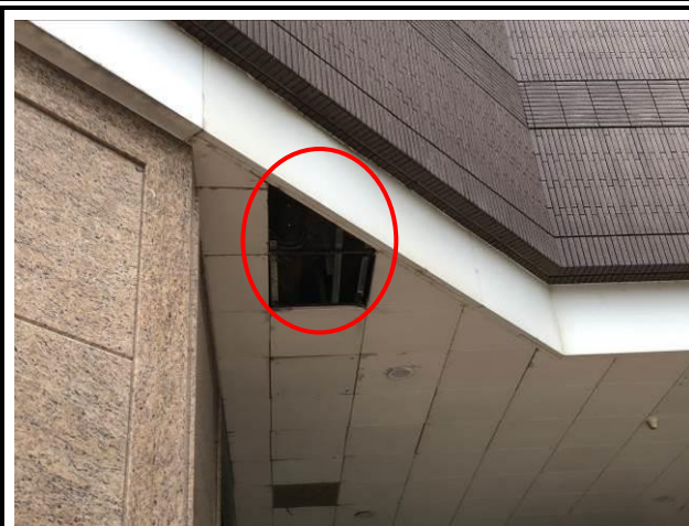
Photo No. B16 2 pieces of ceiling panel were missing
