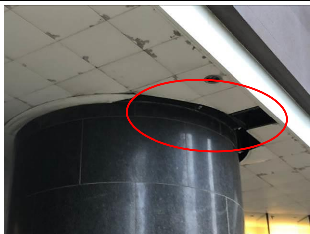
Photo No. B69 | 3 pieces of ceiling panel were missing.
