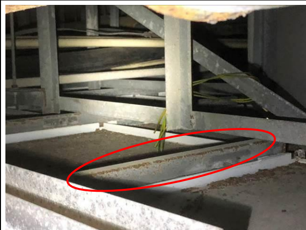
Photo No. B12 | Ceiling grid was rusty.
